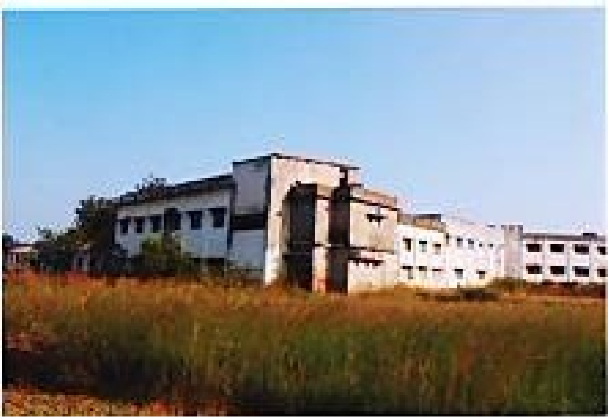
Rear view of the building
