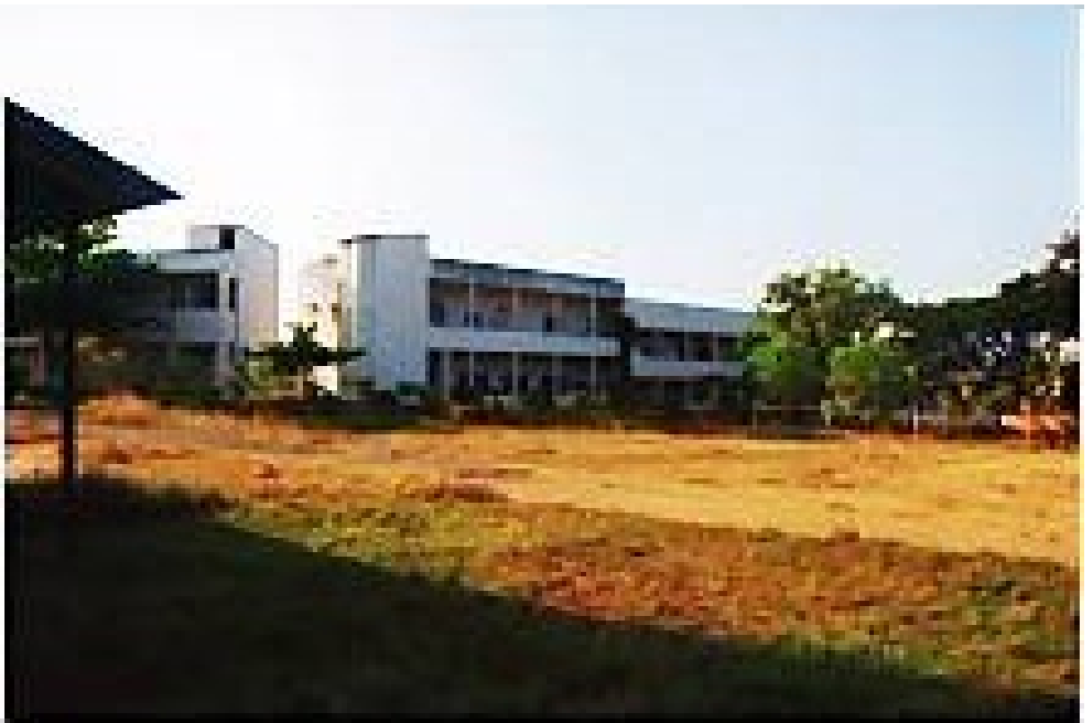
Front view of the Building
